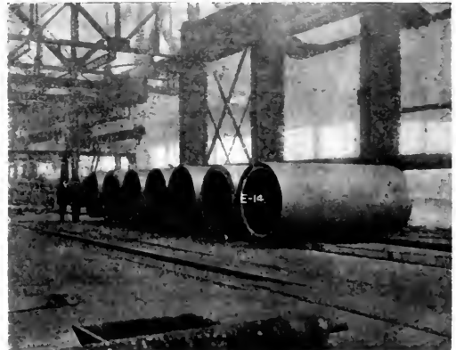
Rough dryer roll castings.
